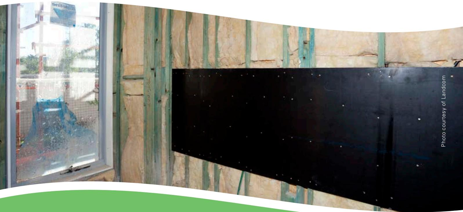
Construction image illustrating reinforcement of walls using sheeting
